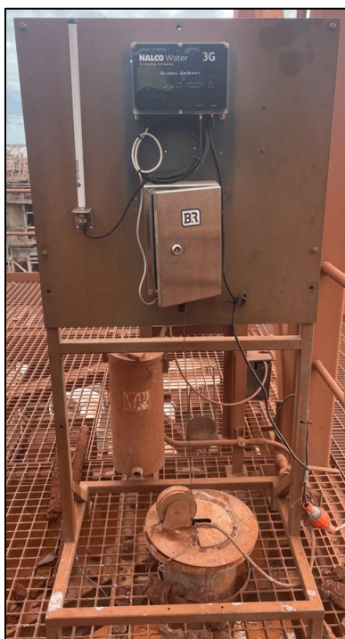
Figure 1. Installed SCRAMO unit on operating washer.
